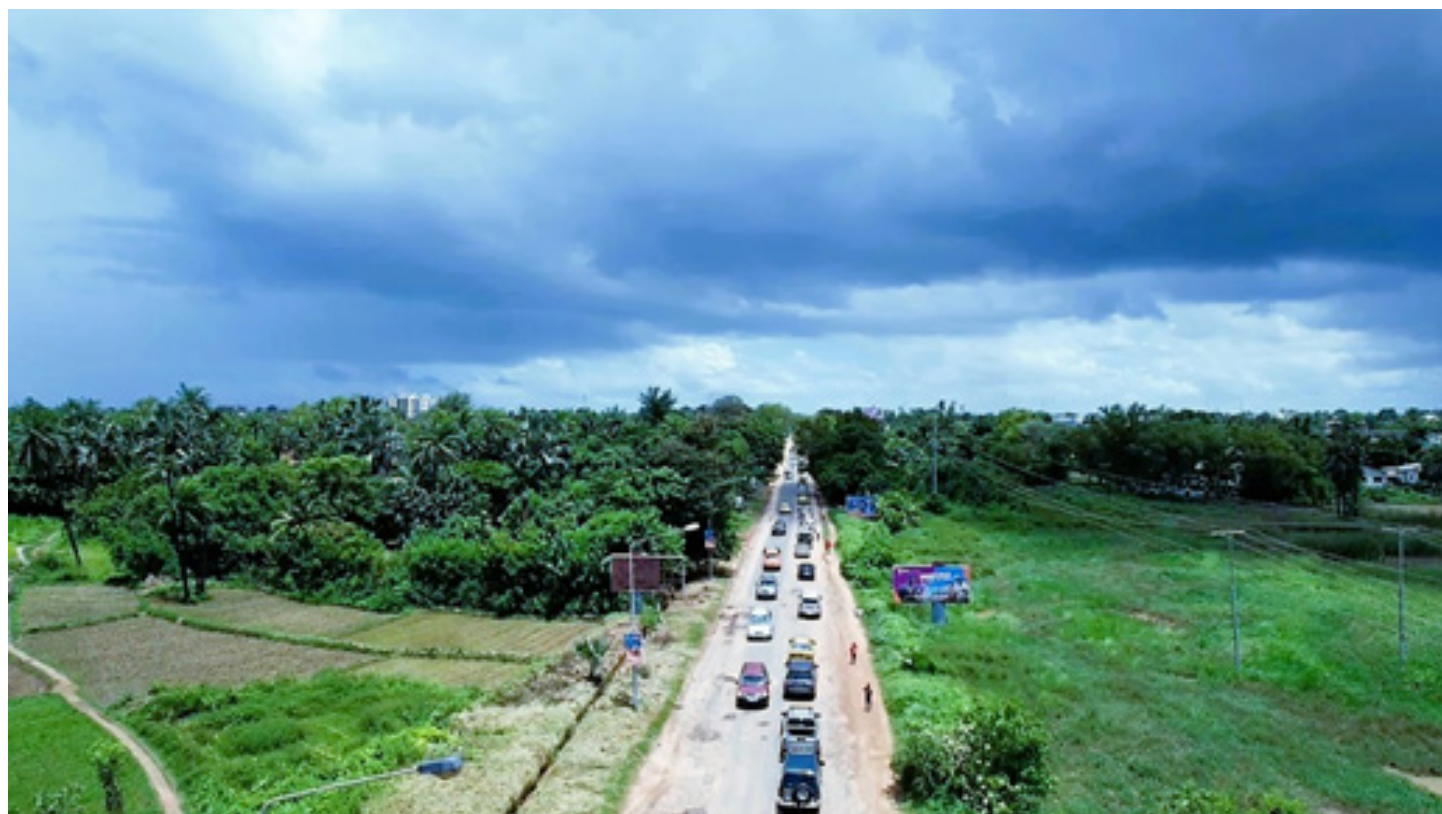
Aerial view of Bertil Harding Highway (2022)
