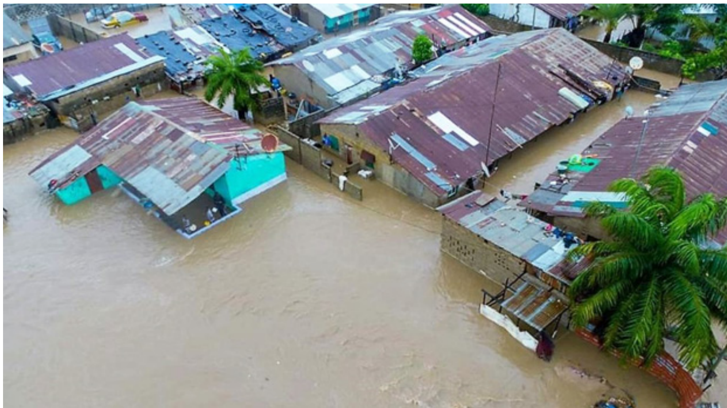
Flooded settlements at Kotu, Kanifing Municipality (2022)
