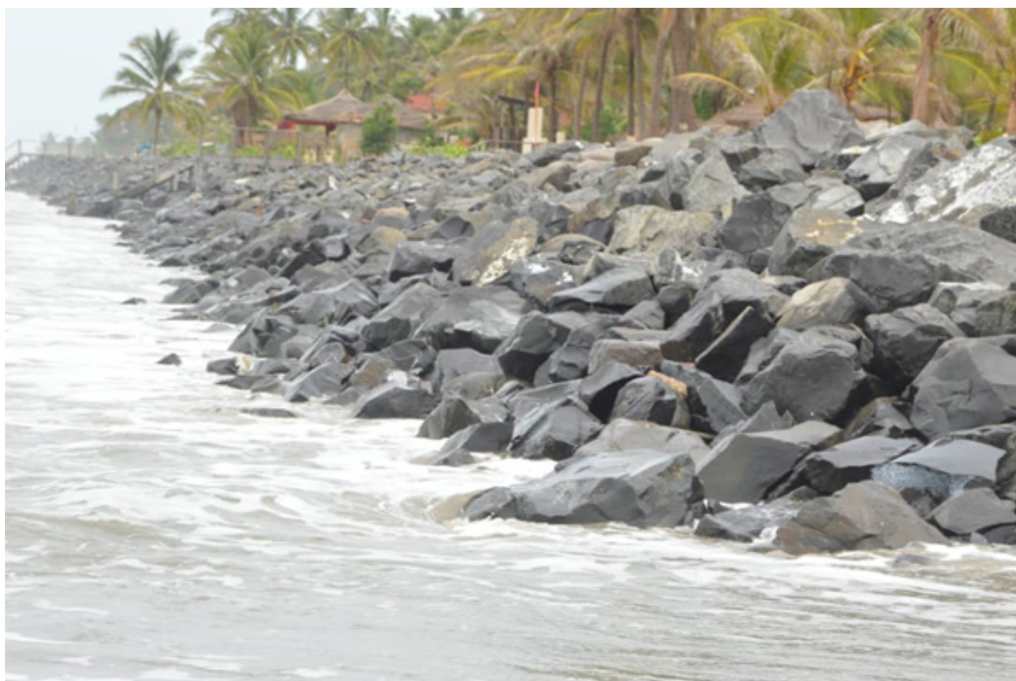
Sea defences against beach erosion to protect a hotel in the Kotu Area (2022)
