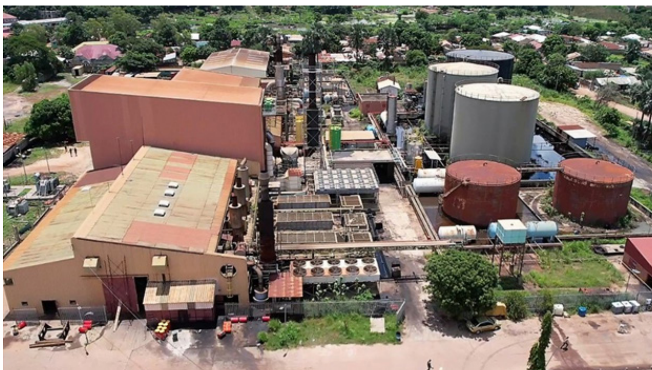
Aerial view of Kotu Power Station, The Gambia's oldest and largest HFO power plant (2022)
